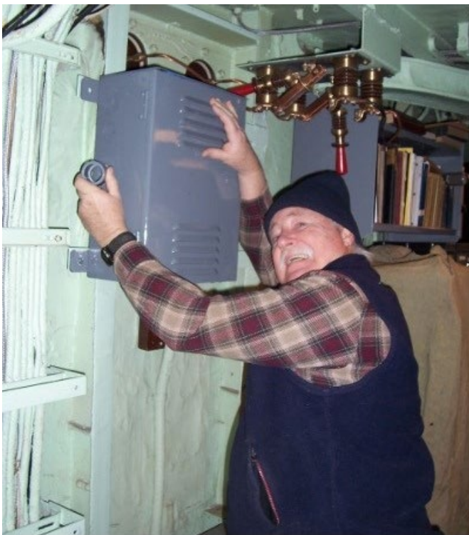
Jerry Jones installing his TBL transmitter filter box.
