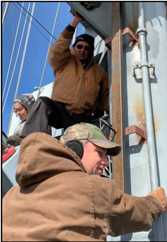
Tim Benner and Matt Clifford working on the wave guide installation
