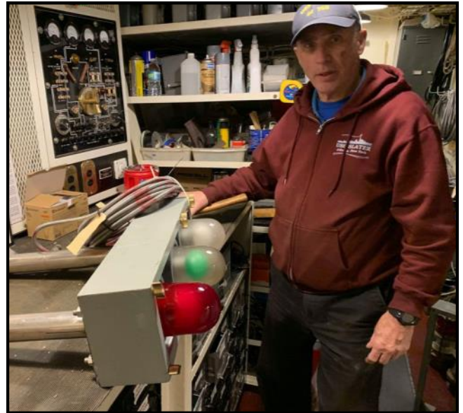
Gary Sheedy wired up the recognition lights that will be installed in the shipyard.
