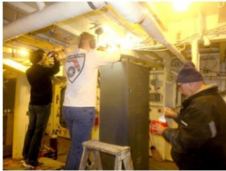
Welding, insulating, and wiring, all going on simultaneously.
