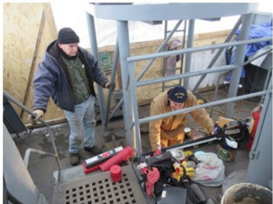
The shipfitters continue to make progress on the flying bridge repairs.
