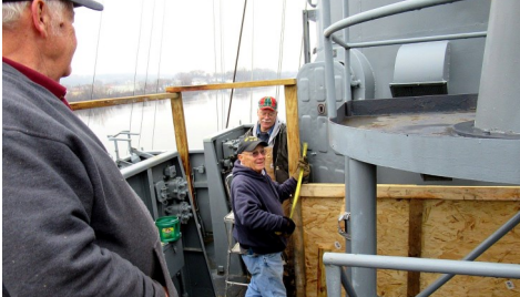
The shipfitters are enclosing the flying bridge for winter work.
