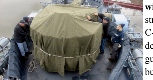
The shipfitters are enclosing the flying bridge for winter work.
