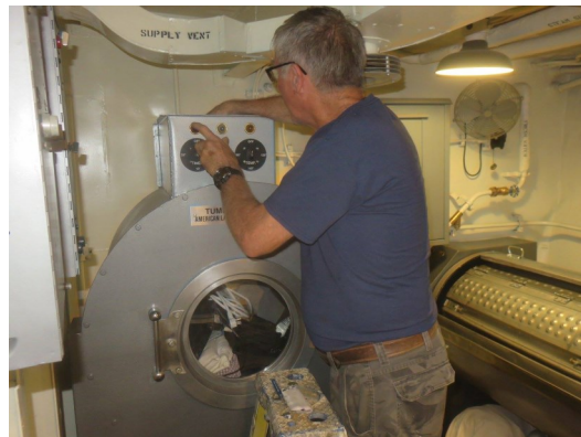
Gary installing new phenolic tags on the laundry dryer.
