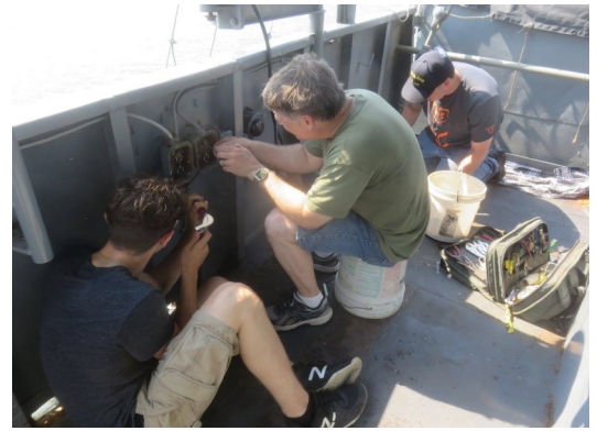
Rewiring the signal lamp, step three. Reconnecting the new cable.
