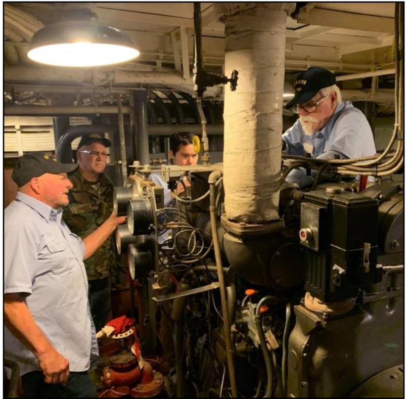
The engineers ran a test of the emergency diesel generator.
