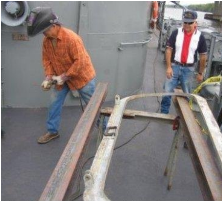
Doug Tanner supervises Laird Confer as they straighten the door frame.
