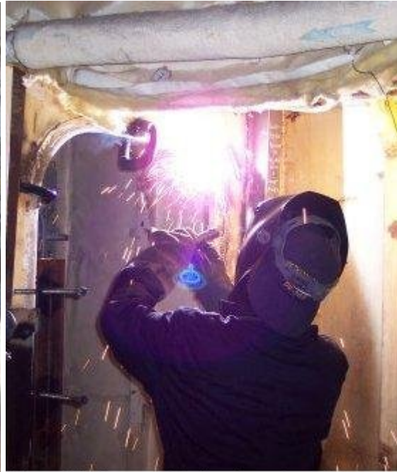
Tom Skufca welds in the door frame.
