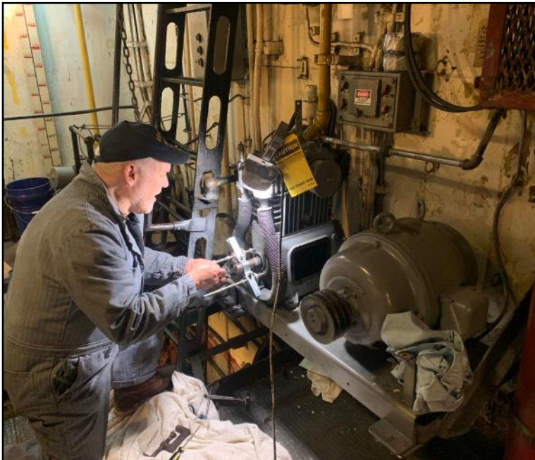
Chuck Tanner, investigating the condition of the Quincy compressor in B-1.
