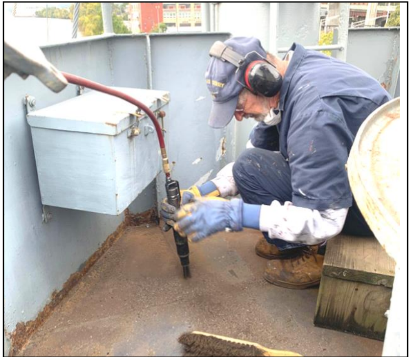
Ron tried to punch more holes on the main battery director platform deck.
