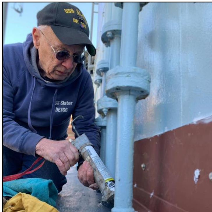
Super Dave Mardon helped seal up that leak in Officer's Country.
