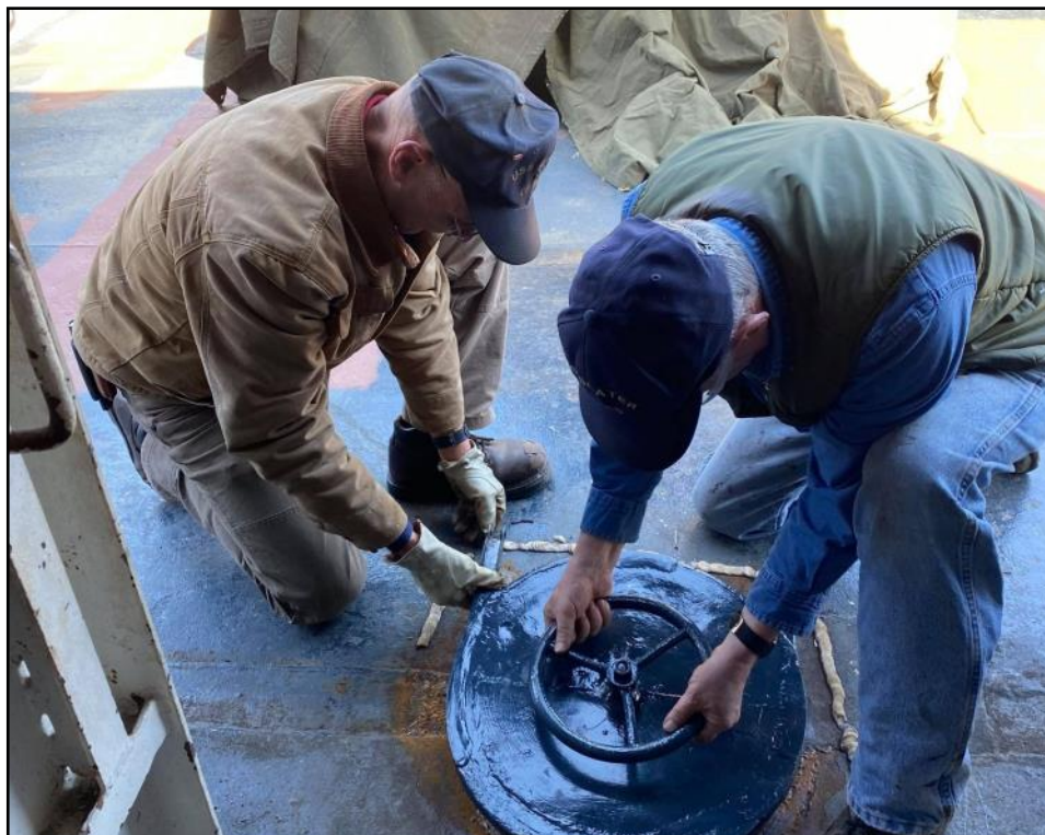
Tim Benner and Chuck Installed the scuttle hatch.
