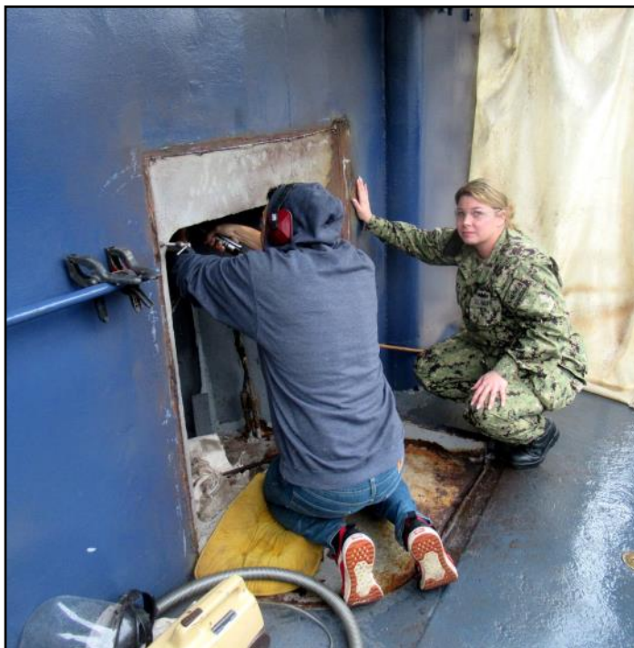
Grinding in the fan room.
