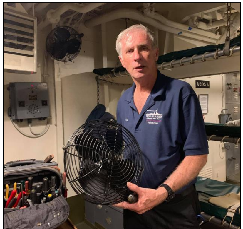
Gary is working on repairing the fans one by one.
