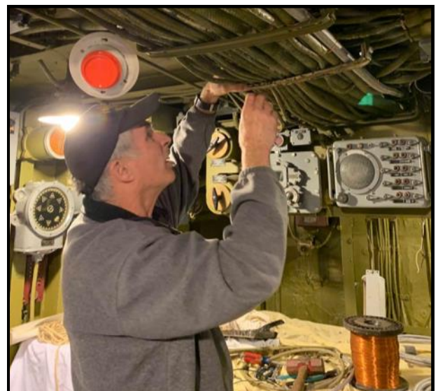
Gary Sheedy, reinstalling cable supports in CIC.
