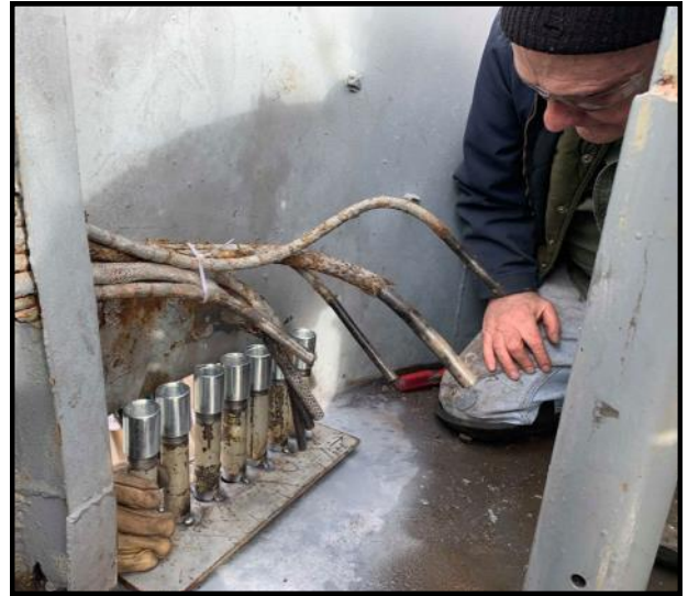
The new stuffing tubes, ready to be welded in.
