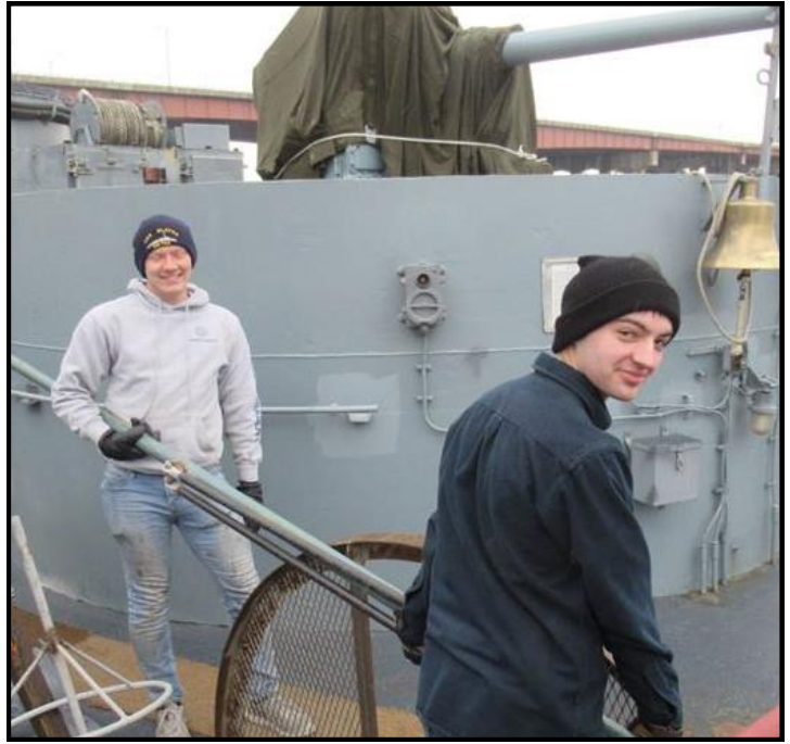
RPI Midshipmen, Branden and Jack, staged the new mast part by the gangway for blasting and painting.
